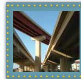
Overpass $7 million per lane mile
